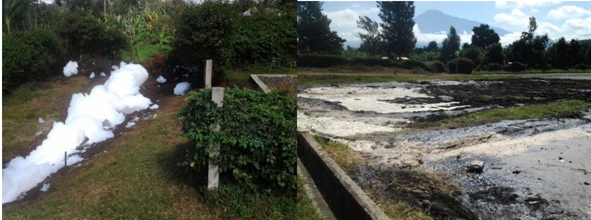
Figure 3.20 Photos taken in August 2013 at the Arusha Municipal Sewage Treatment System showing evidence of industrial effluent.
